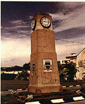
First War Memorial Monument built at Padanggan Road in 1951.
