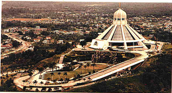
The Building of Dewan Bandar Kuching Utara (Kuching City North)
