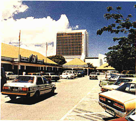
Petra Tunku Building, Miri
